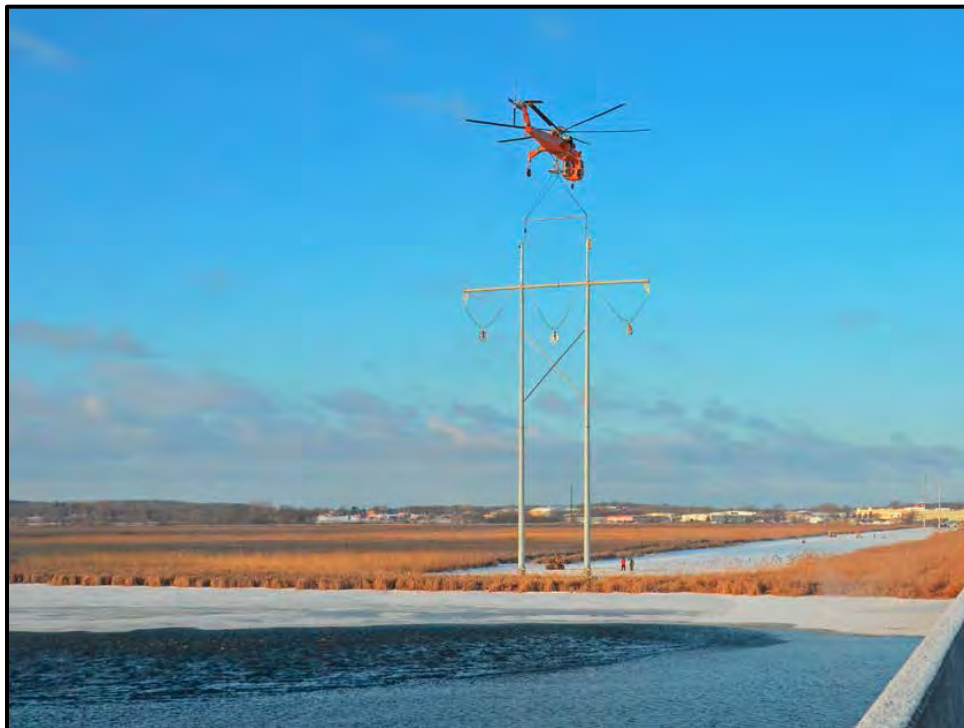
Figure 2.4-13. Installing a structure on a foundation with a helicopter.
