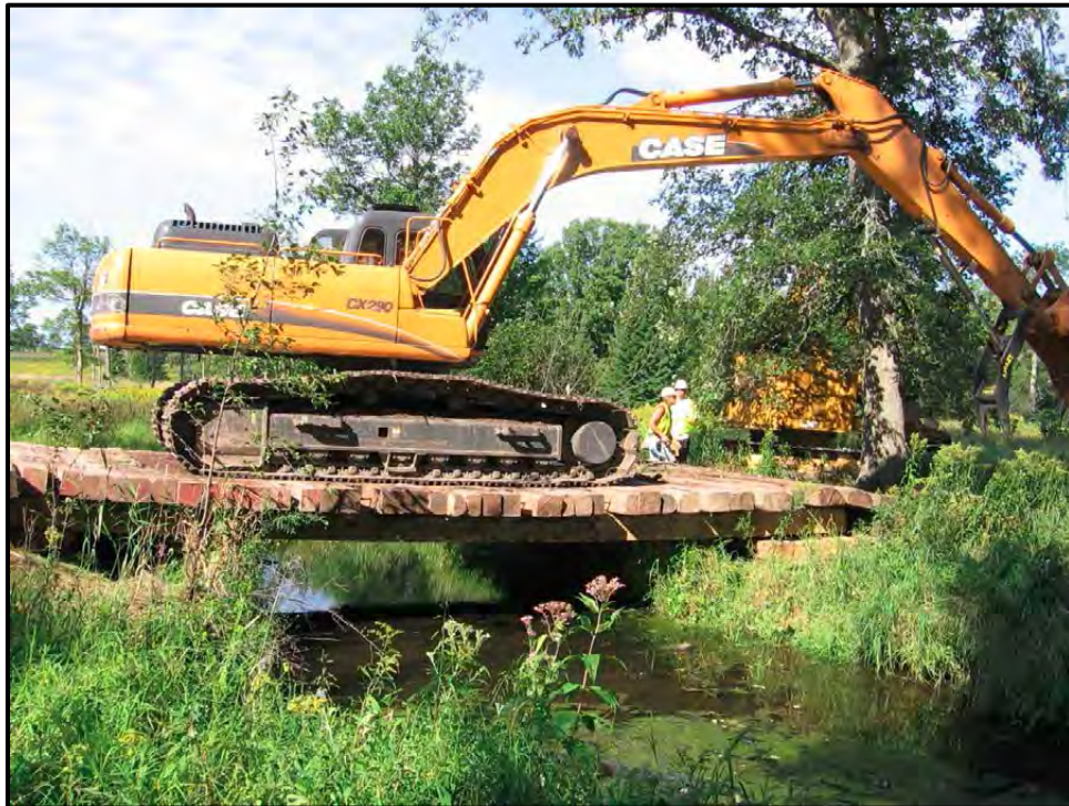
Figure 2.4-9. Timber-mat equipment bridge at a stream crossing.
