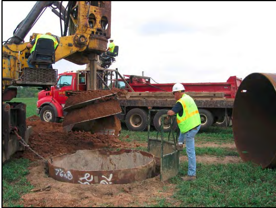
Figure 2.4-10. Foundation excavation using an auger in dry upland soils.
