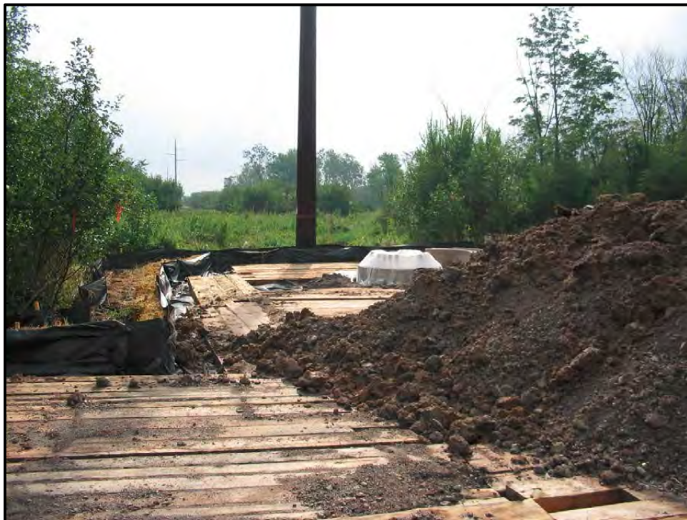
Figure 2.4-11. Structure location in a wetland—matted work platform, foundation, spoil pile (to be removed), and erosion control.
