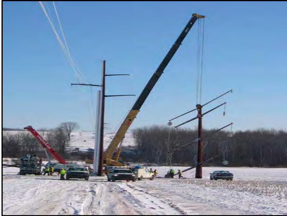
Figure 2.4-12. Installing the top section of a structure with a crane.
