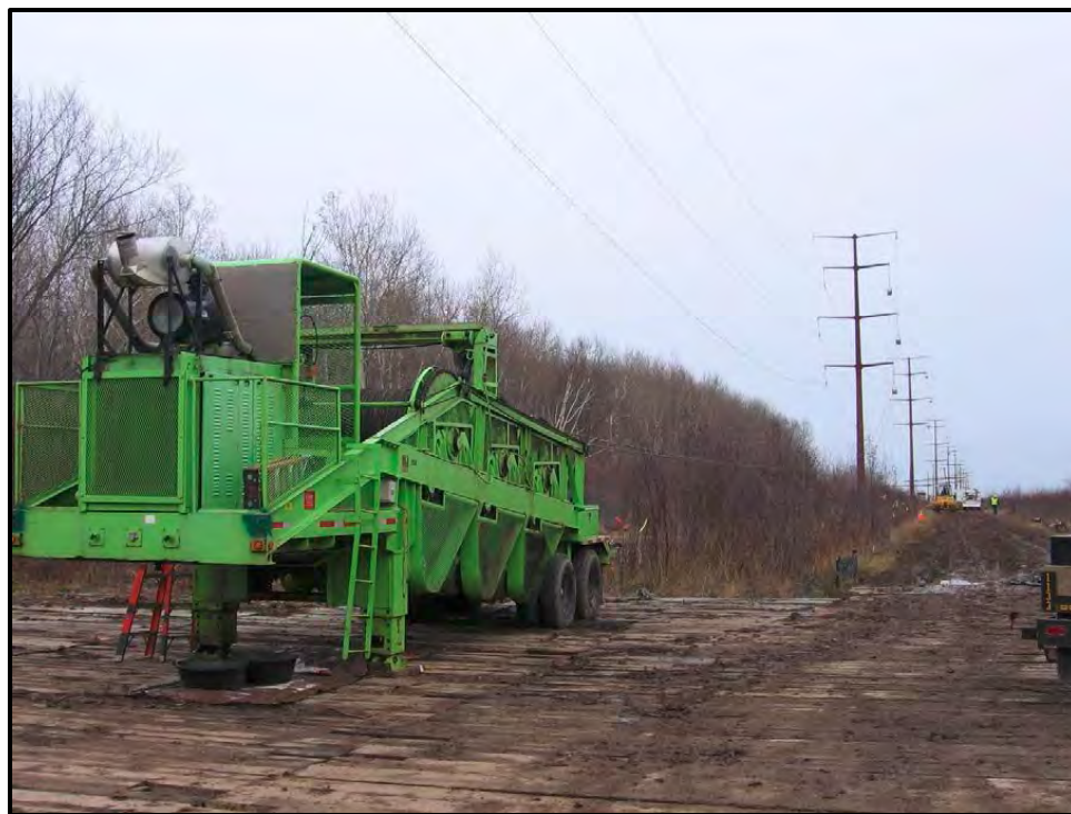
Figure 2.4-14. Pulling the conductor through the structure arms.
