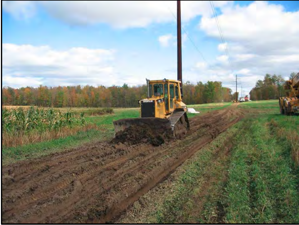
Figure D.4. Ruts being smoothed with blade.
