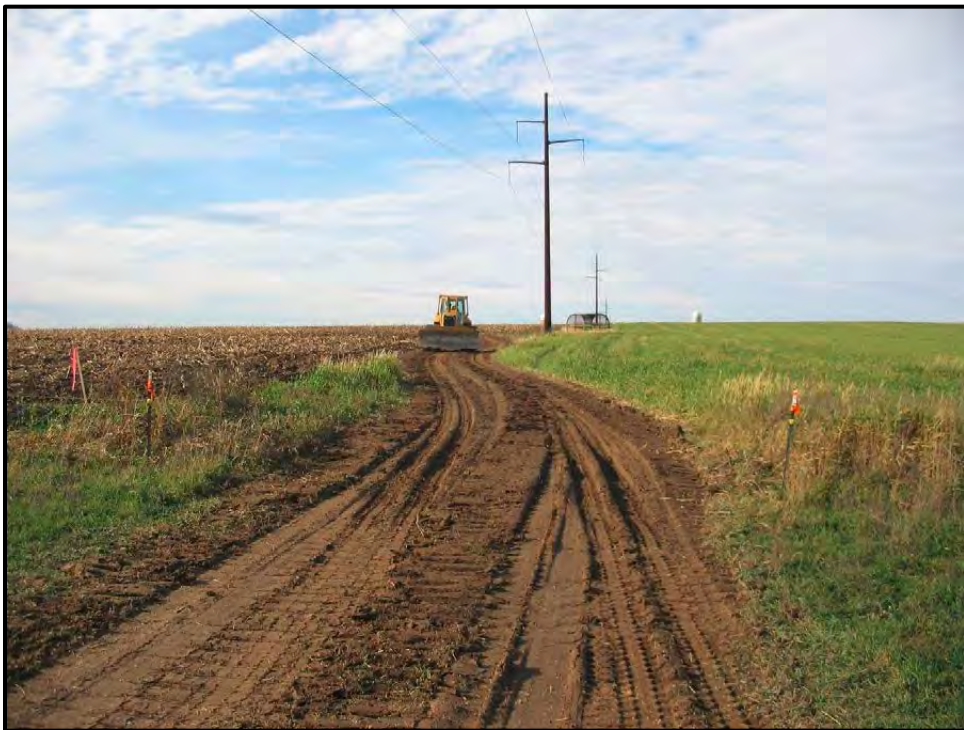
Figure D.5. Smoothing out ruts by backblading with a dozer.
