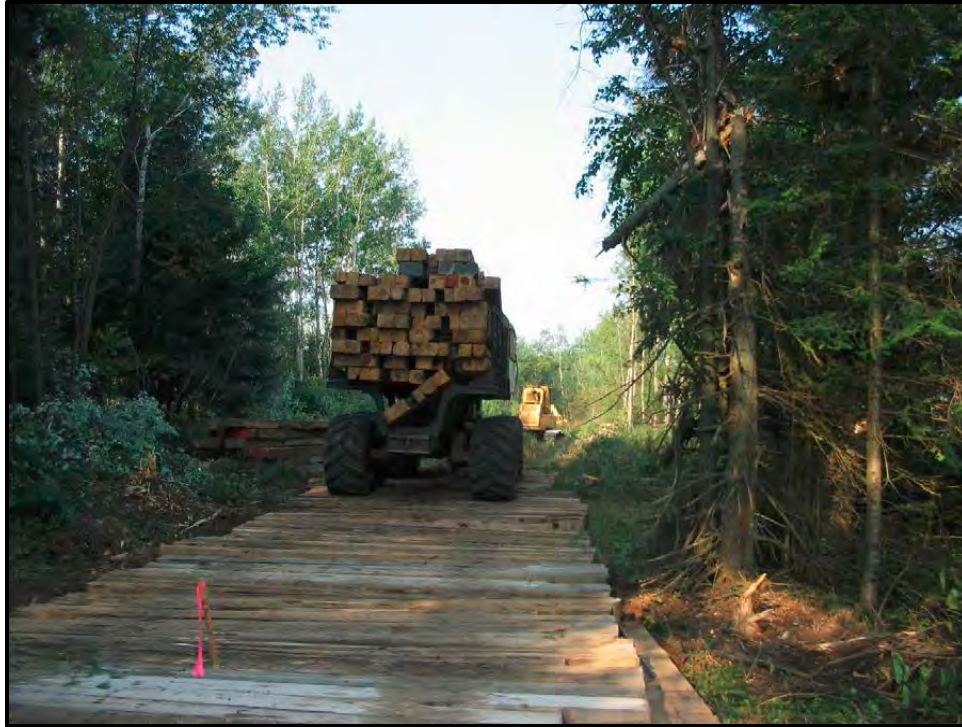
Figure D.9. Timber mats being placed in wooded wetland.
