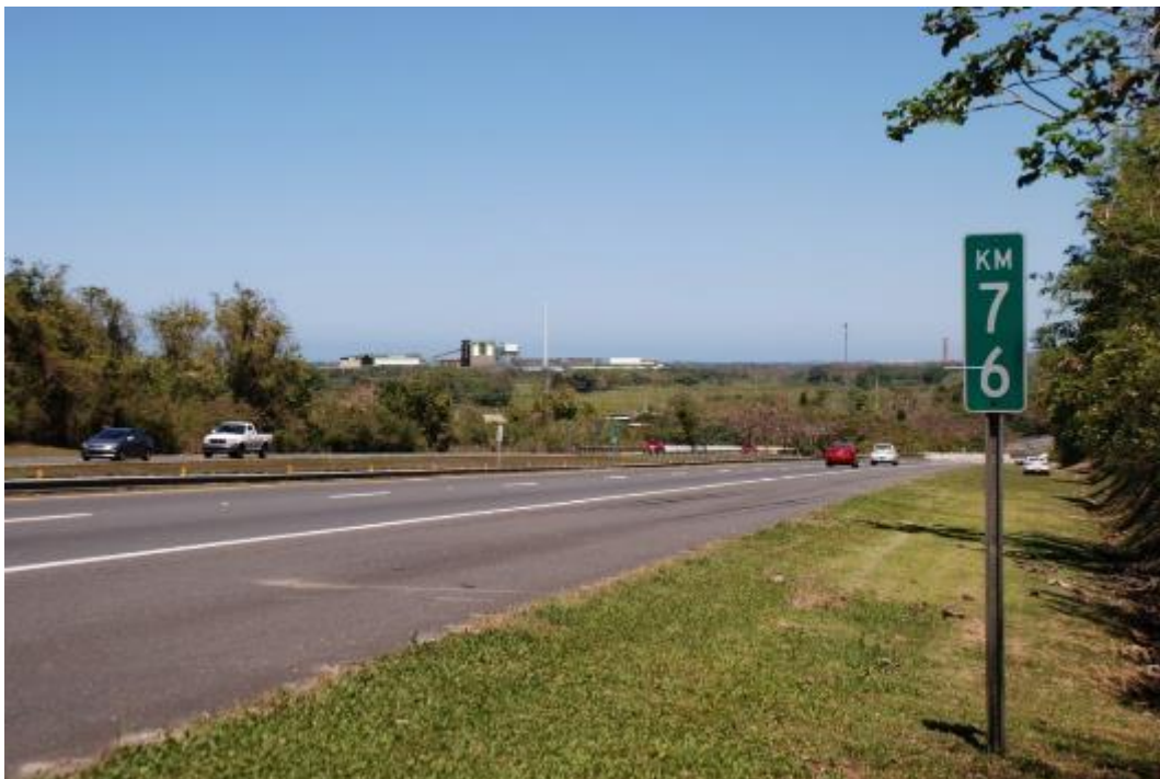
Figure B-10b. Key Observation Point 7 – Photosimulation of Project Site from Highway PR-22
