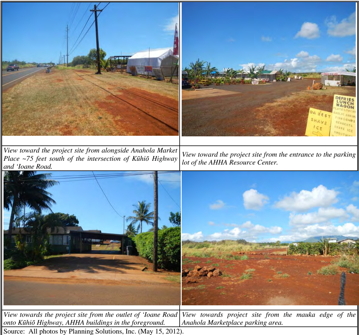
Figure 5.13. Views Near the Intersection of Kūhiō Highway and ‘Ioane Road
