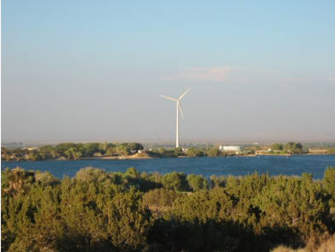
Figure 2-5. Palmdale Water District On-Site Wind Turbine
