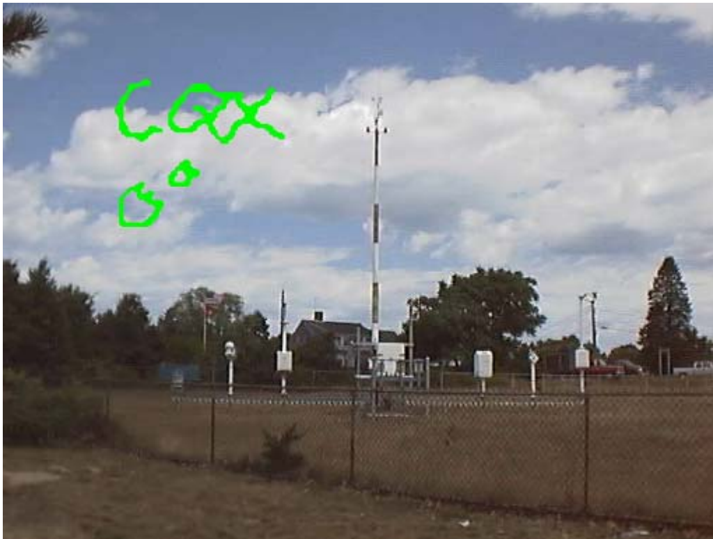
Figure 4-9. Chatham Municipal Airport Met Tower (from NOAA web site).
