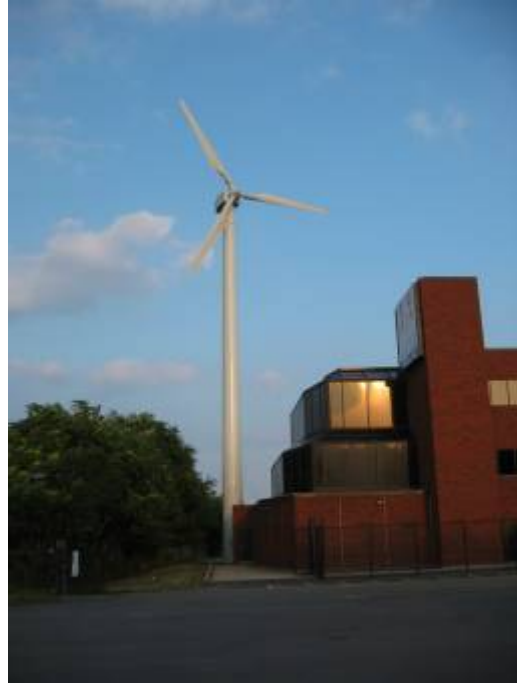
Figure 2-7. IBEW Wind Turbine
