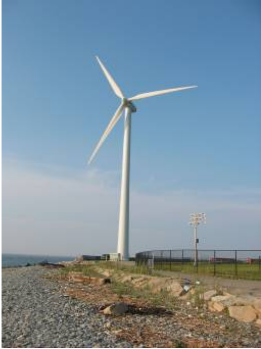
Figure 2-6. Hull 1 Wind Turbine
