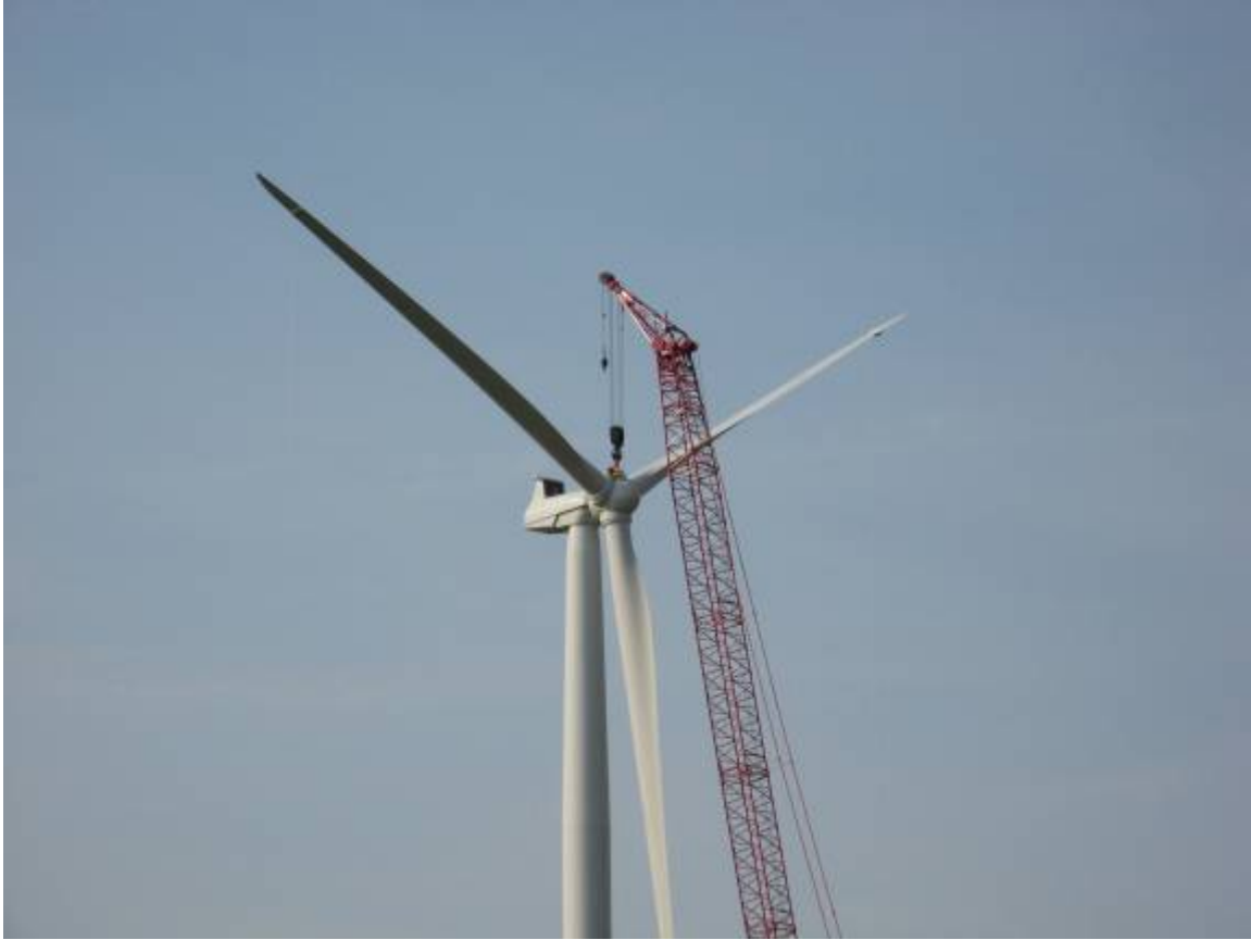
Figure 2-3. Installation of a Vestas V82 in Northern Michigan
