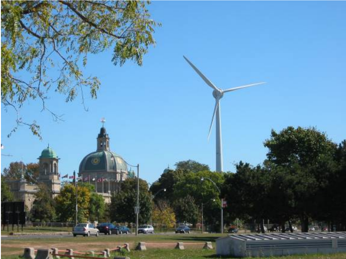
Figure 2-8. Wind Turbine at Toronto's Exhibition Place
