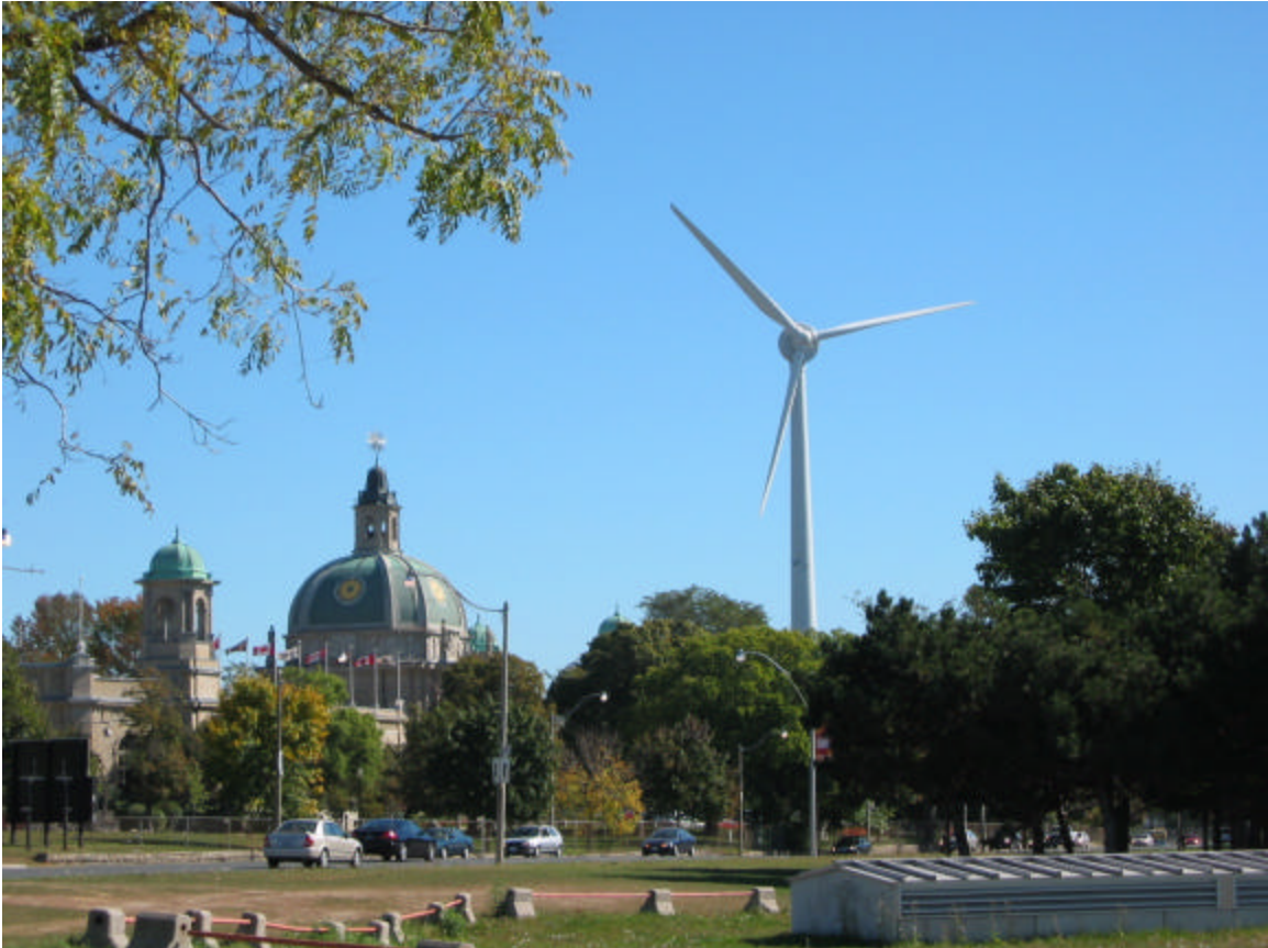
Figure 2-8 Wind Turbine at Toronto's Exhibition Place
