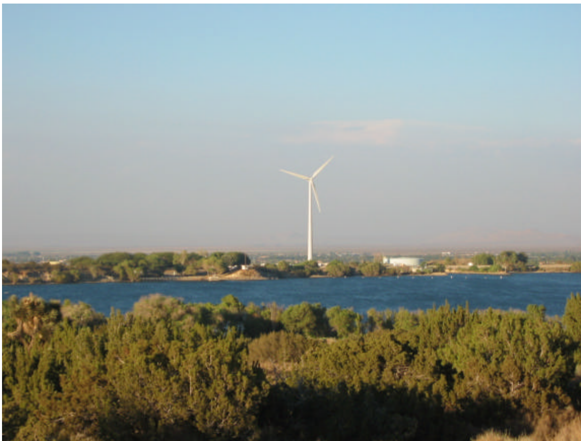
Figure 2-5 Palmdale Water District On-Site Wind Turbine
