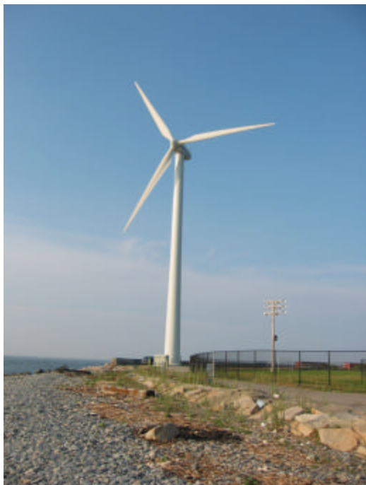
Figure 2-6 Hull 1 Wind Turbine
