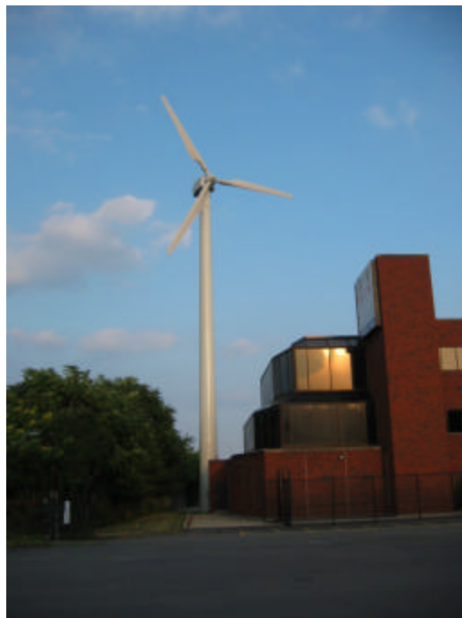
Figure 2-7 IBEW Wind Turbine
