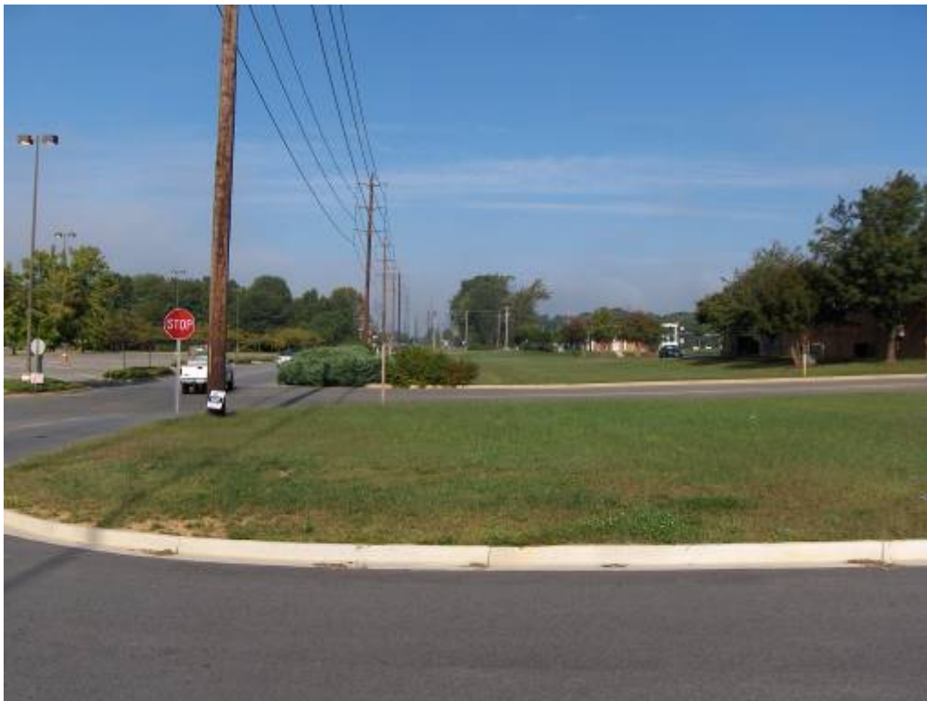
Pole Location 222 Facing West.
