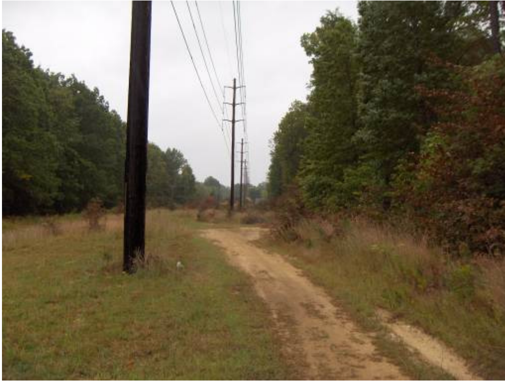
Pole Location 229 Facing East.
