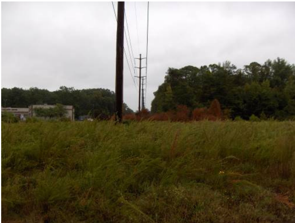
Pole Location 230 Facing East.
