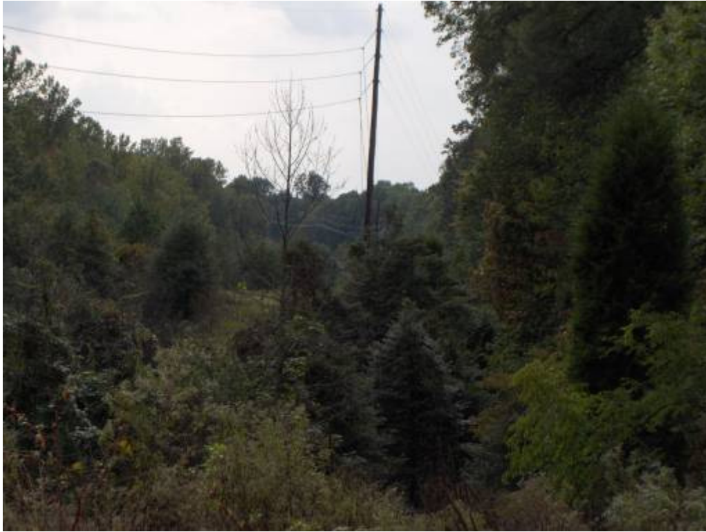
Pole Location 213 Facing Southwest
