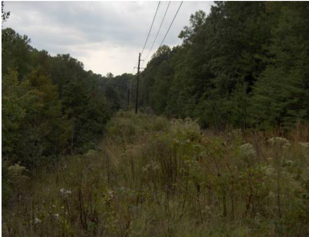
Pole Location 212 Facing Southwest.
