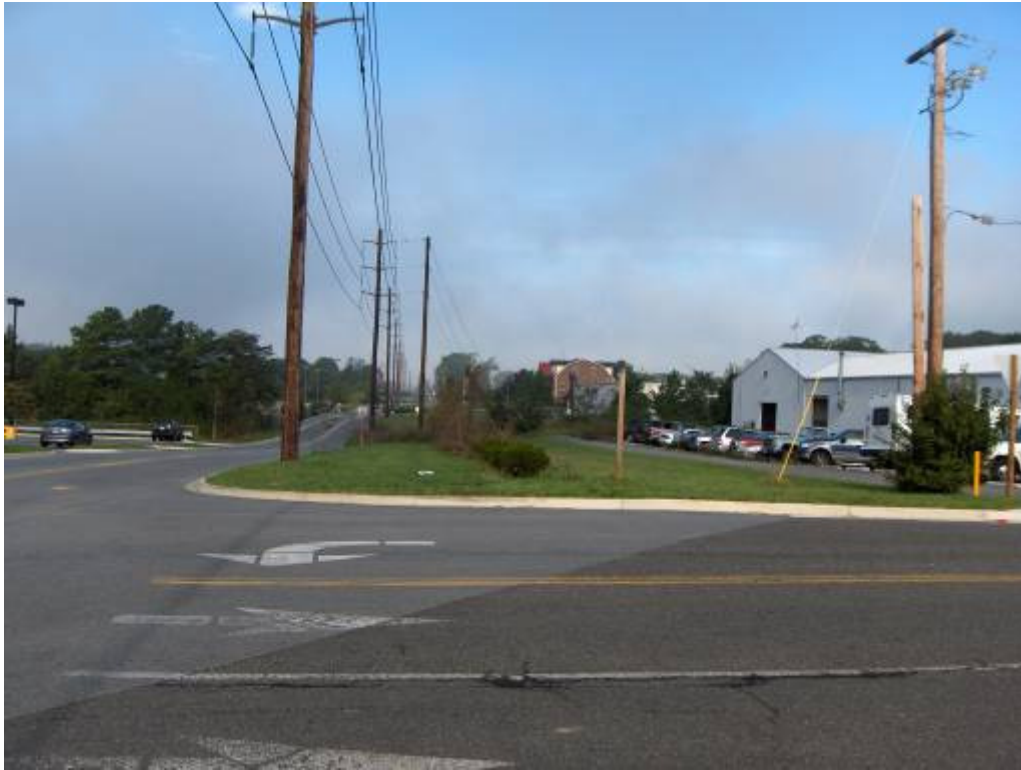
Pole Location 223 Facing West.
