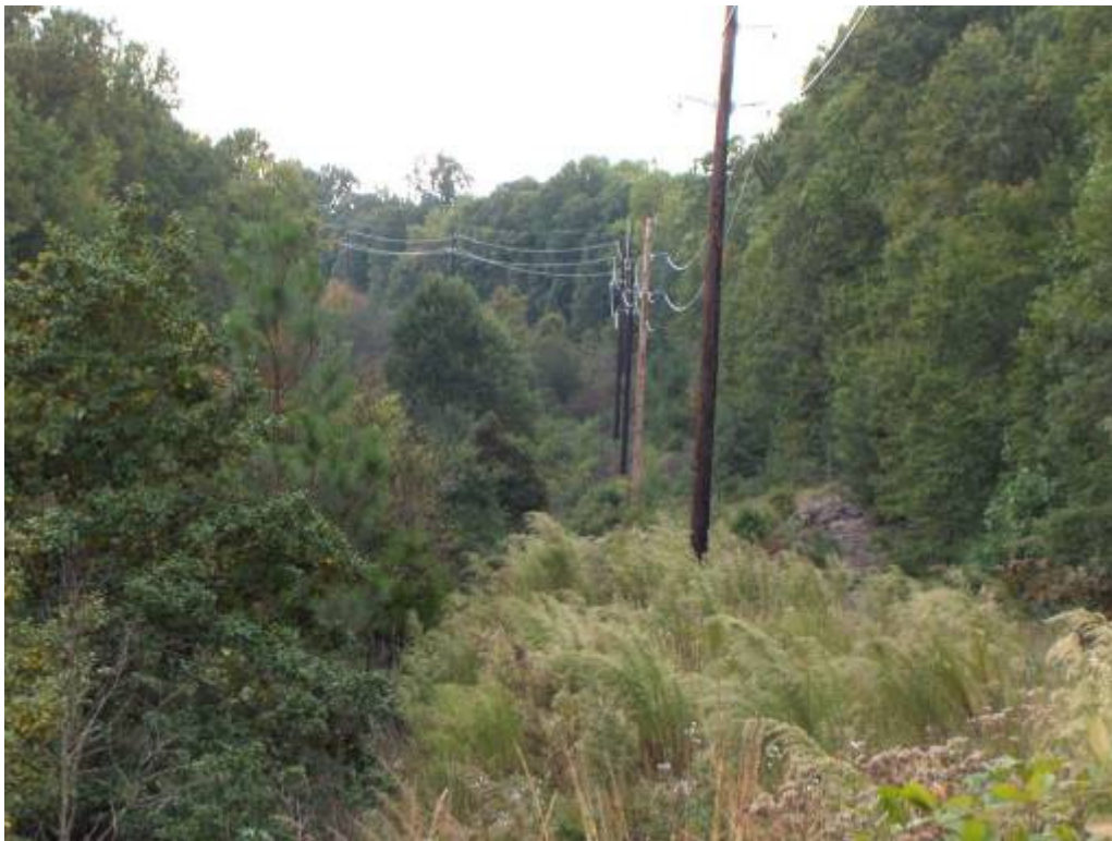
Pole Location 214 Facing Southwest.
