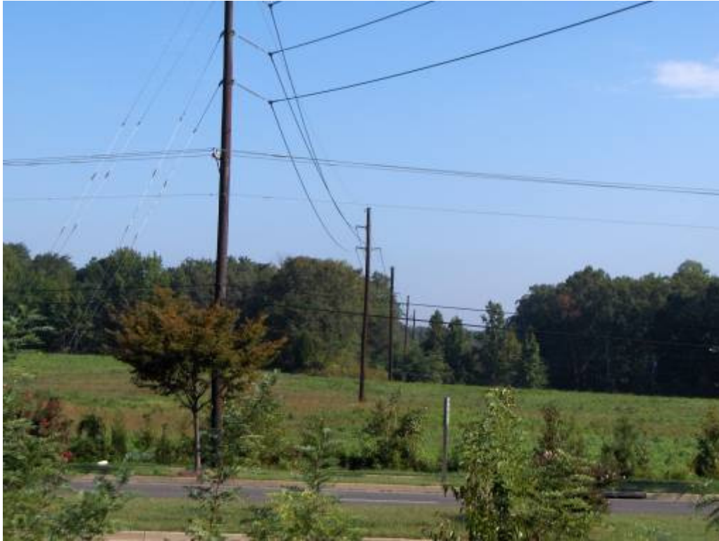
Pole Location 219 Facing North.
