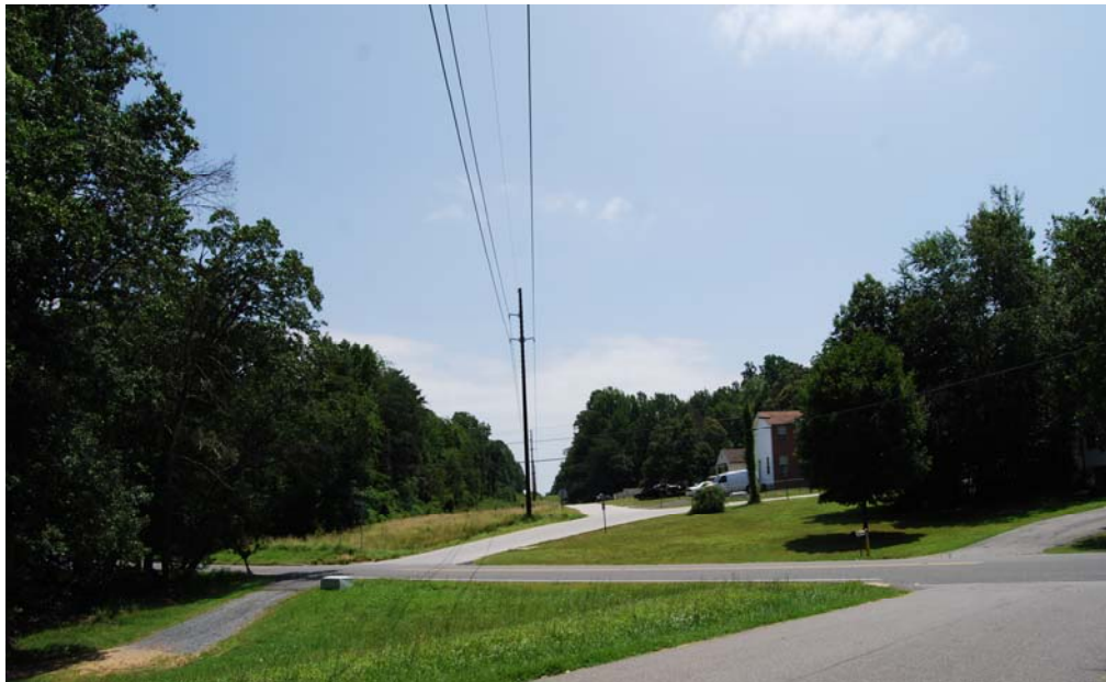
Figure 1-3 The Current SMECO 69 kV Line in the White Sands Neighborhood Source: Black & Veatch
