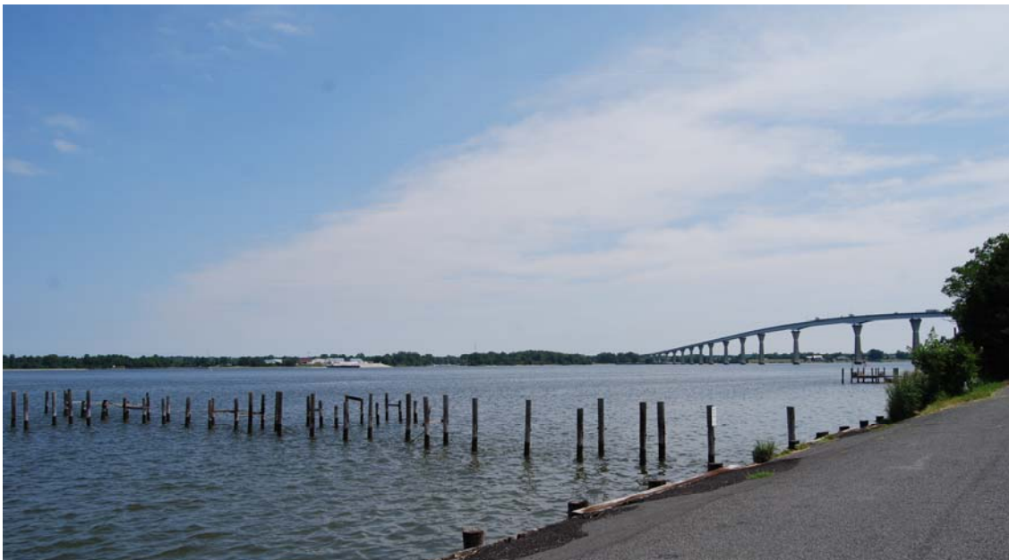
Figure 1-5 The Memorial Bridge River Crossing (taken from St. Mary's County) Source: Black & Veatch
