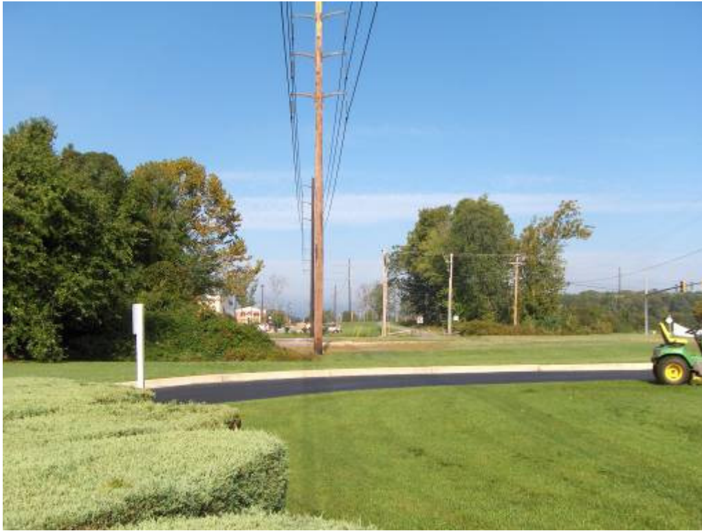
Pole Location 221 Facing West.
