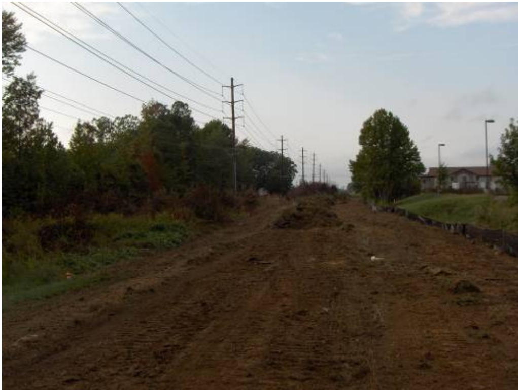
Pole Location 226 Facing West.
