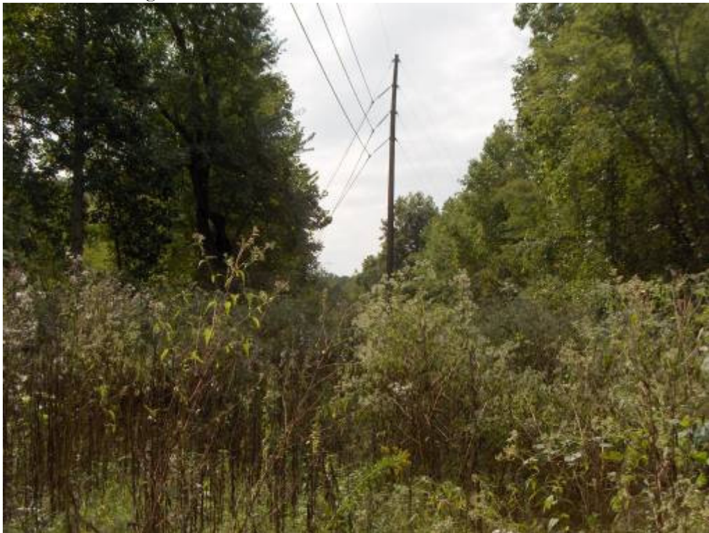
Pole Location 204 Facing Southwest.
