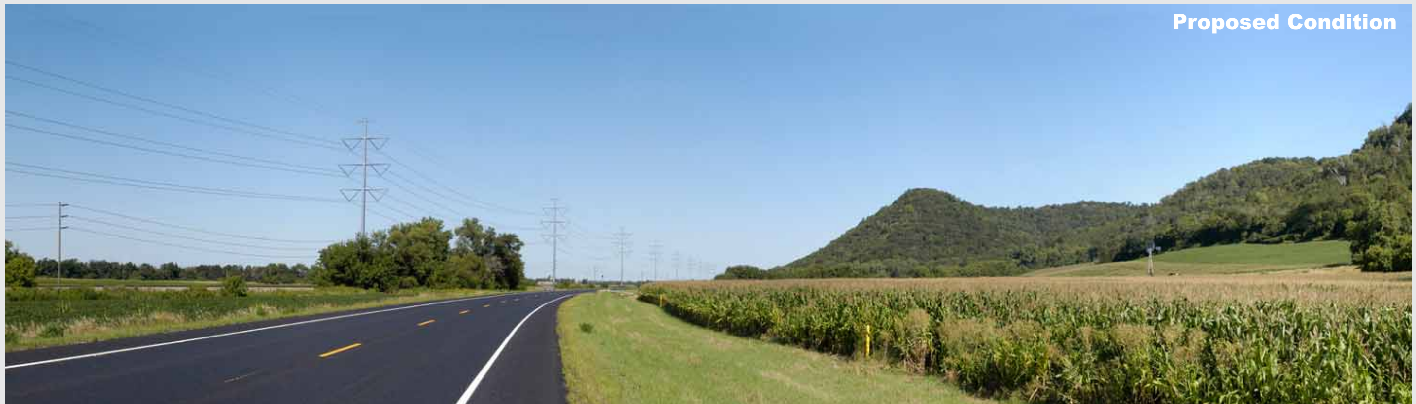
Photopoint 166 - 1.5 miles south of Cochrane, looking northwest. Proposed 345 kV line and existing Dairyland 161 kV consolidated west of road with existing Xcel 69 kV. Dairyland 69 kV removed. The proposed consolidates all transmission lines along the Great River Road.
