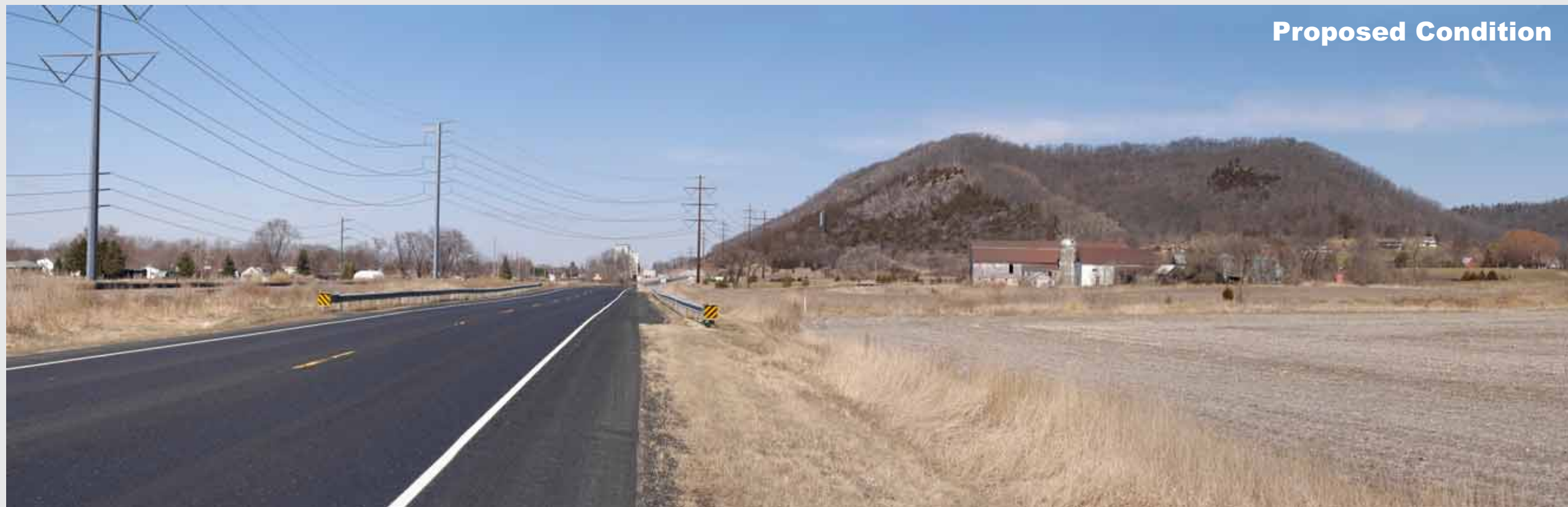
Photopoint 65 - One-half mile south of Cochrane looking northwest. The existing Dairyland Q1 161 kV transmission line would be removed from the Scenic Easement area on the bluff side of the GRR and rebuilt as a double-circuit 161 / 345 kV transmission on the River side of the GRR where no scenic easements exist.
