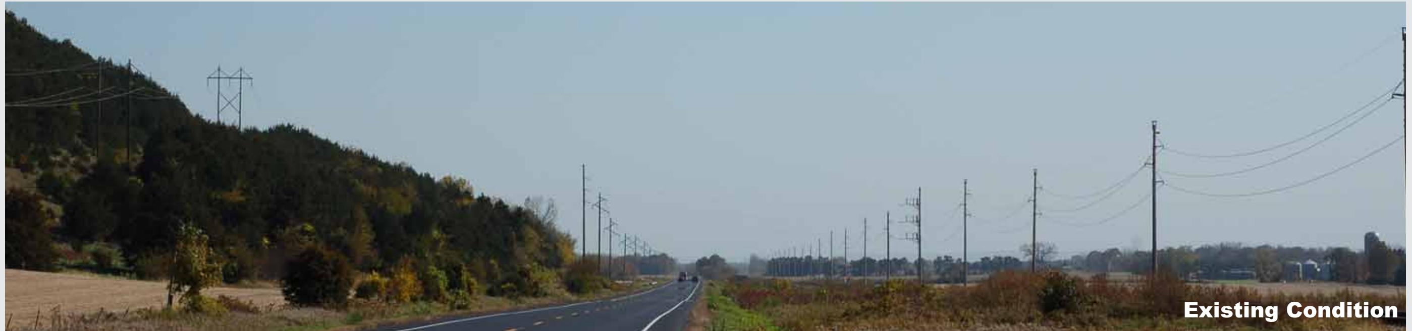
Photopoint 191 - 0.25 mile southwest of Wisconsin St., Cochrane. Looking Southwest. Three existing transmission lines along Great River Road: 161 kV on far left, 69 kV on left side of road, 69 kV on far right.
