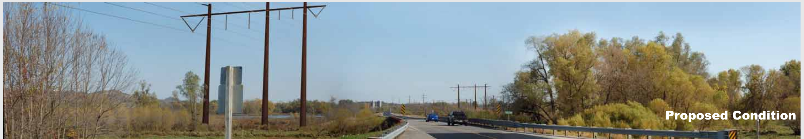
Photopoint 192 - 0.4 miles east of Trempealeau River. Looking west. H-frames requested by WisDOT to reduce height and visual impact. Also see Photopoint 64.
