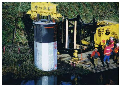
Helicopter Based Vibratory Caisson and Hammer Unit
