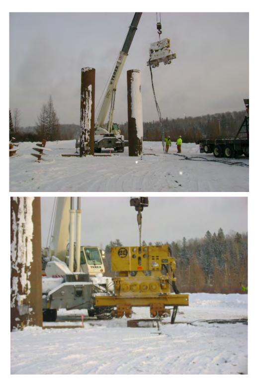
Ground Based Vibratory Caisson and Hammer Unit
