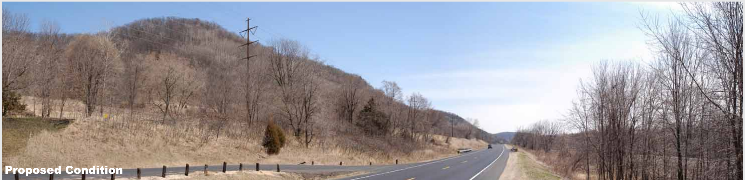
Photopoint 76 - Bluff side pull out, 1.5 miles south of Dairyland's Alma power plant. Looking southeast. Existing Dairyland 161 kV line rebuilt to 345 / 161 kV double circuit on left side of photo paralleling Great River Road. Designed specifically to allow screen of trees to remain.
