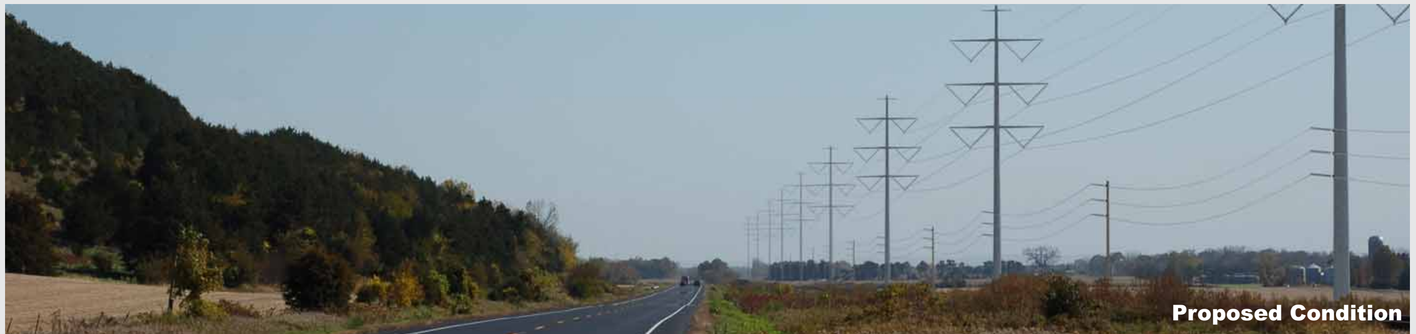
Photopoint 191 - 0.25 mile southwest of Wisconsin St., Cochrane. Looking Southwest. The existing Dairyland Q1 161 kV transmission line would be removed from the Scenic Easement area on the bluff side of the GRR and rebuilt as a double-circuit 161 / 345 kV transmission line on the River side of the GRR where no scenic easements exist. In the distance, the route follows the railroad and would remove existing transmission lines from the GRR.
