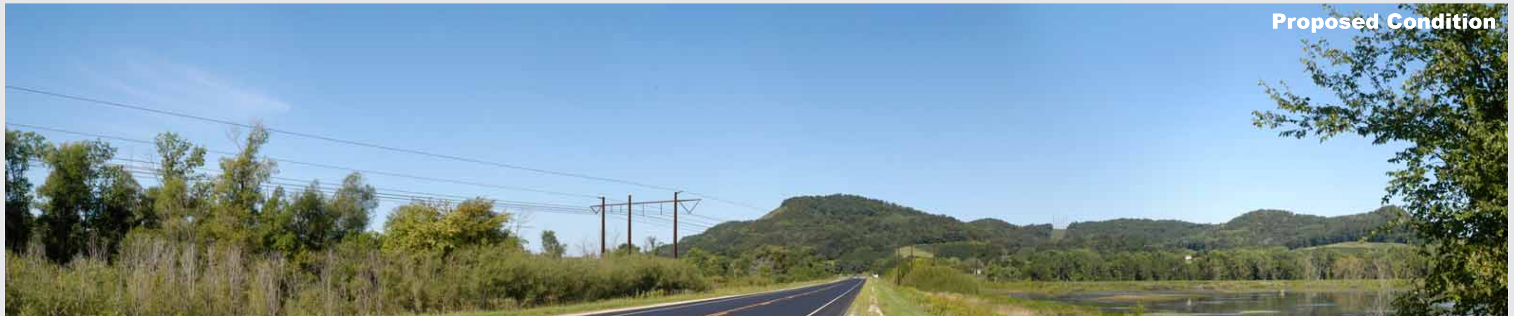
Photopoint 64 - Trempealeau River Bridge east of Marshland. Leaf on condition in winter. Looking West. Existing Dairyland 161 kV line rebuilt to 345/161 kV double circuit. Shorter H-frame poles reduce visual impacts of road crossing.
