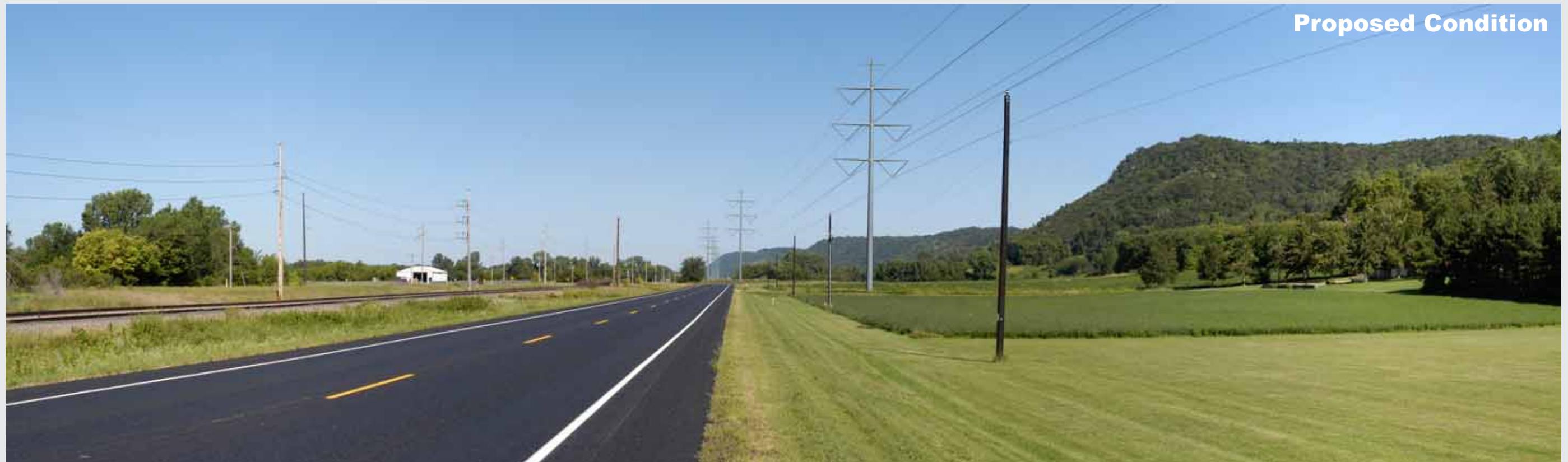
Photopoint 169 - 1 mile north of Cochrane, looking northwest. Existing Dairyland Q1 161kV transmission line would be rebuilt as a double circuit 161 / 345 kV transmission line.
