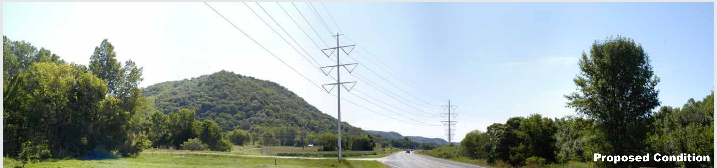
Photopoint 174 - 2.0 miles southeast of Dairyland's Alma power plant, looking southeast. The existing Dairyland Q1 161 kV transmission line would be rebuilt as a double-circuit 161 kV / 345 kV transmission line.
