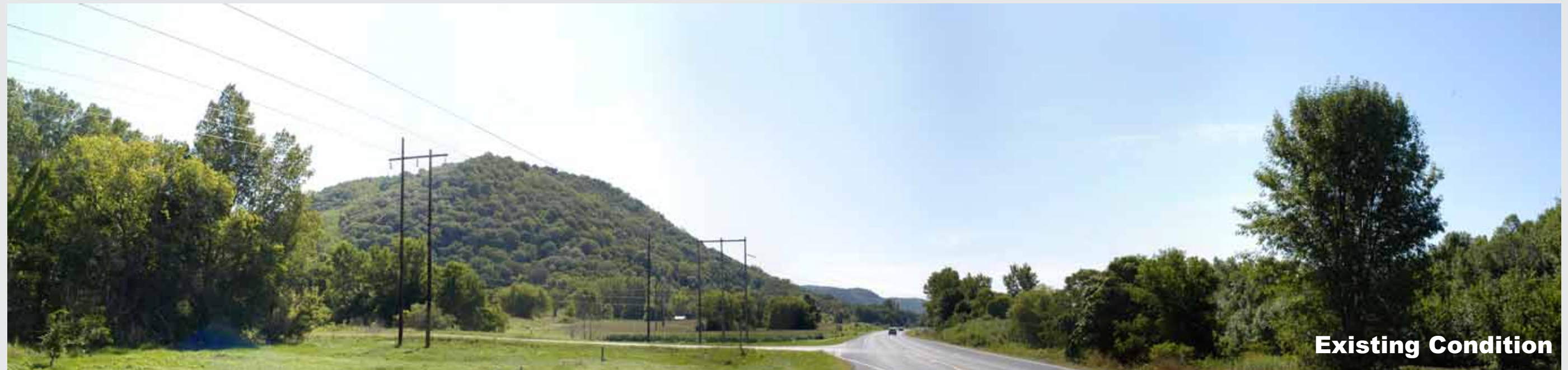
Photopoint 174 - 2.0 miles southeast of Dairyland's Alma power plant, looking southeast. The existing Dairyland Q1 161 kV transmission line crosses the Great River Road (WIS 35) at the Dairyland Power Road intersection.
