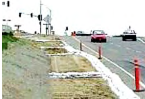
Photo 1.0: Sand Bag Barrier
