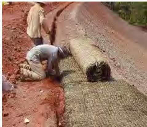
Photo 1.0: Erosion Control Blanket Application
