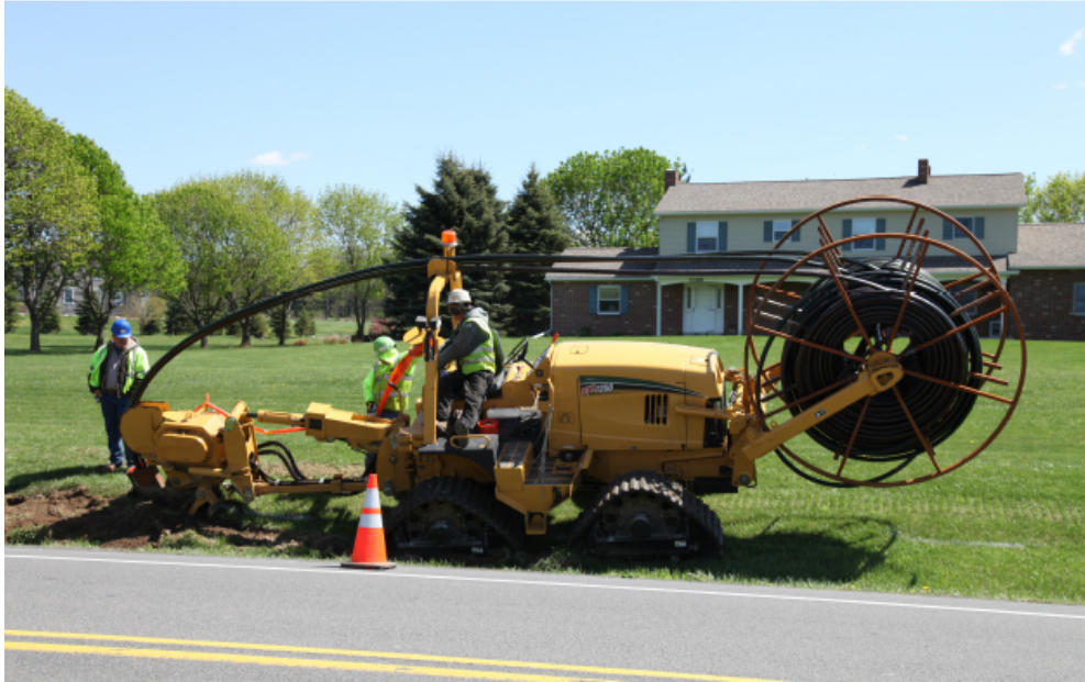
Figure 2-4. Vibratory plowing along a roadway. Source: Power and Communication Contractors Association
