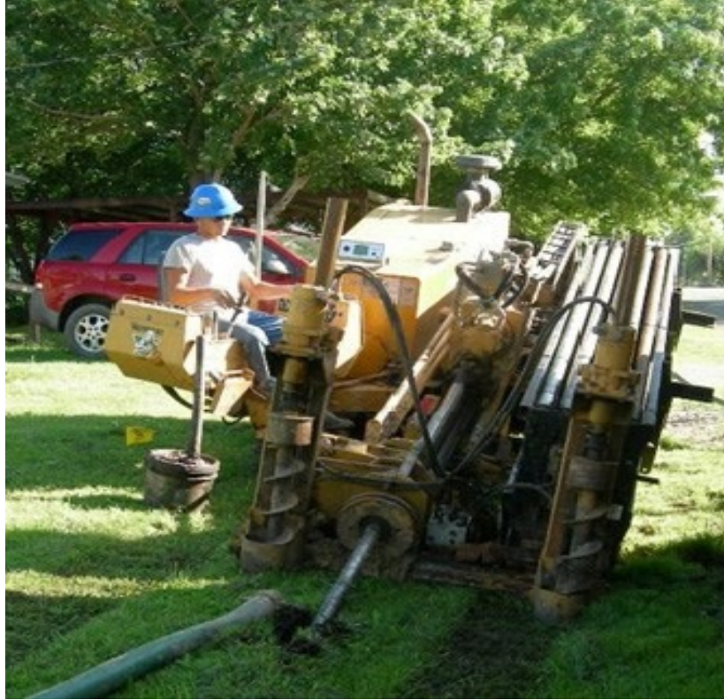
Figure 2-6. Directional Boring Machine. Source: The Fiber Optic Association
