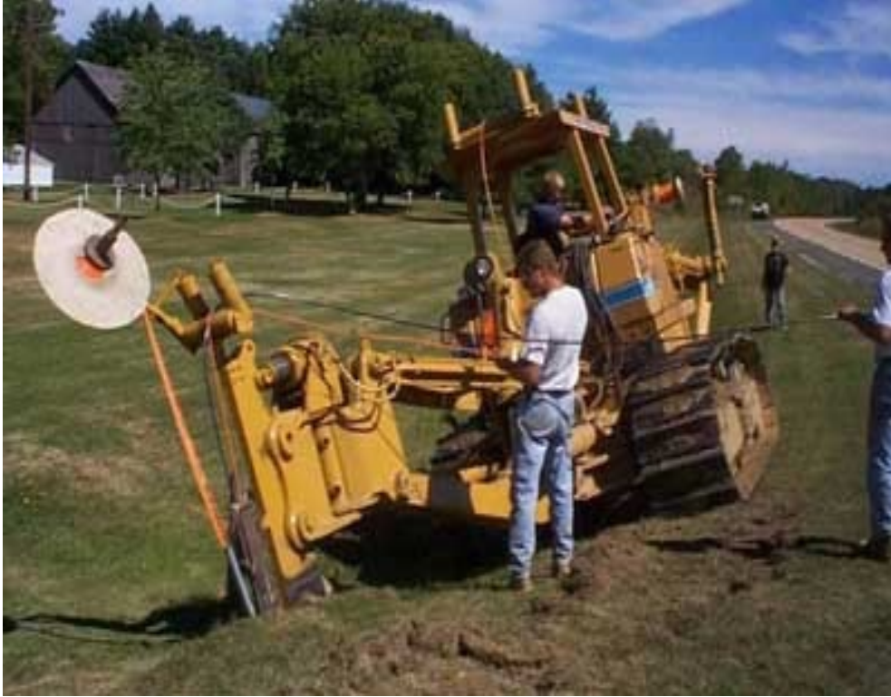
Figure 2-2. Plowing Method of Installation Source: The Fiber Optic Association
