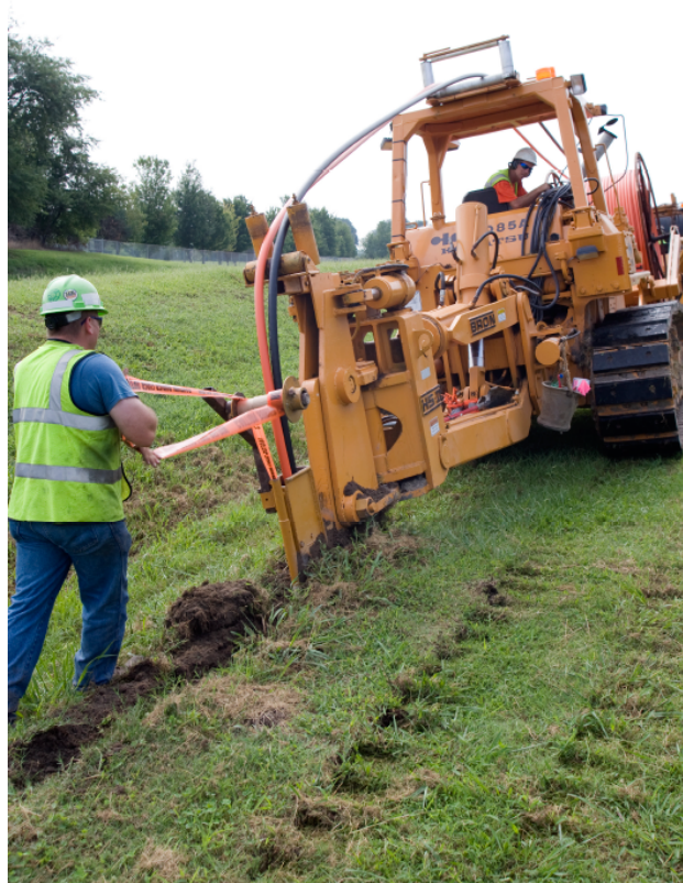
Figure 2-3. Plowing along a roadside. Source: Power and Communication Contractors Association
