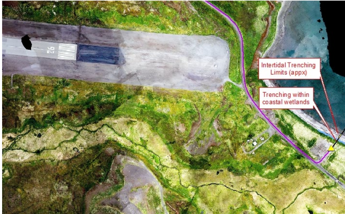
Figure 64. Cold Bay Landfall Conditions Aerial
