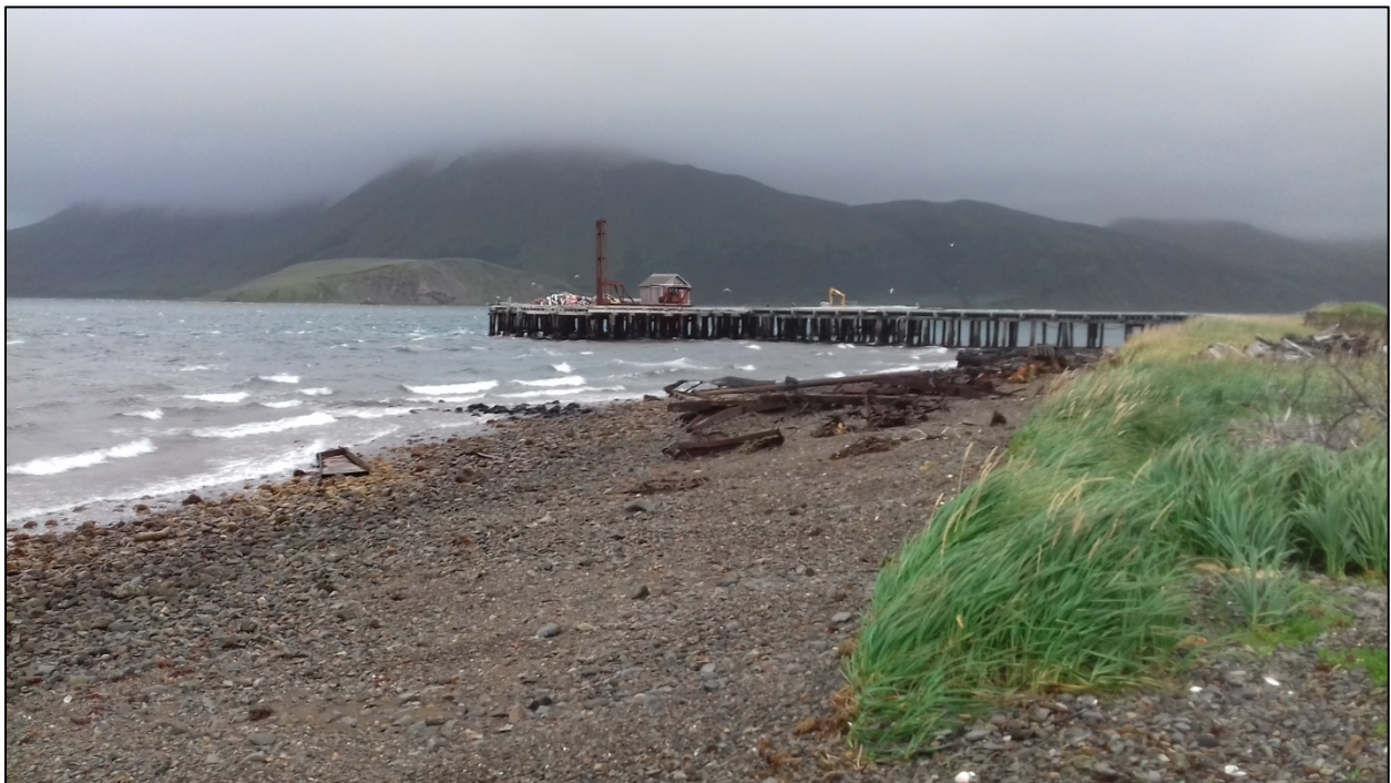
Figure 68. False Pass Landfall Existing Conditions Facing the Peter Pan Dock
