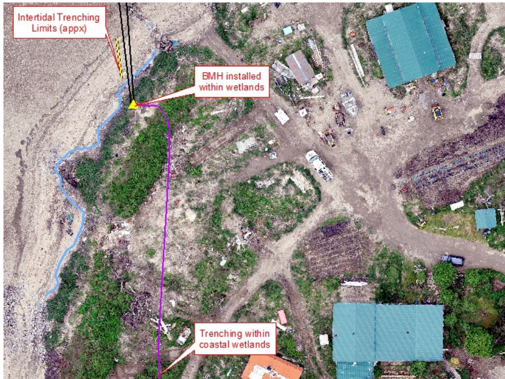
Figure 52. Chignik Lagoon Landfall Existing Conditions Aerial
