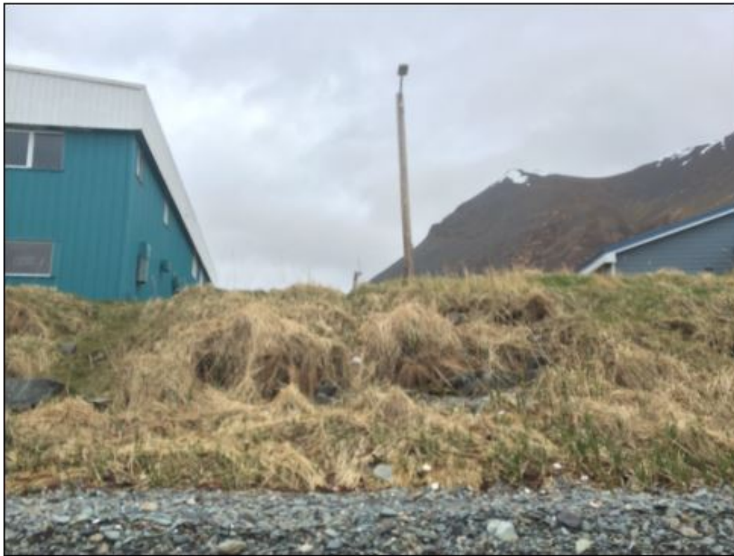
Figure 62. King Cove Landfall Existing Substrates facing BMH
