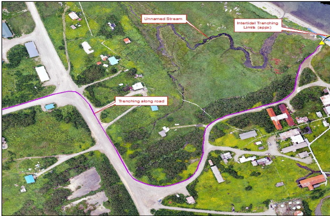
Figure 67. False Pass Landfall Existing Conditions Aerial
